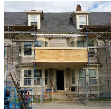
Highland Avenue, Hardwick
