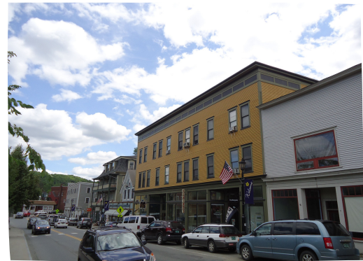
Bemis Block in Hardwick is anchored at street level by commercial business space. Apartments for older renters and renters with disabilities are located upstairs.
